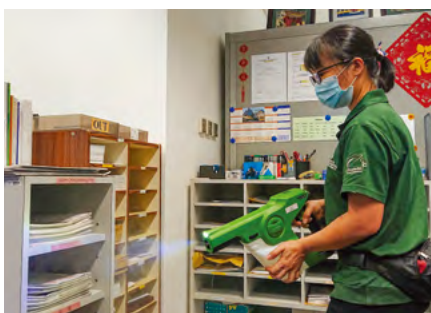
Anti-microbial coating is applied to faculty offices and the department office.
